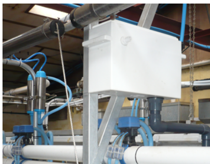
HEADER TANK (Note: Level With Cylinders)
