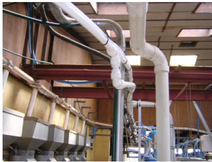
FLEXIBLE PIPE RUN
