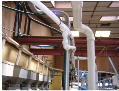
FLEXIBLE PIPE RUN
