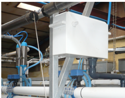
HEADER TANK (Note: Level With Cylinders)
