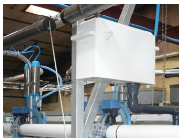
HEADER TANK (Note: Level With Cylinders)
