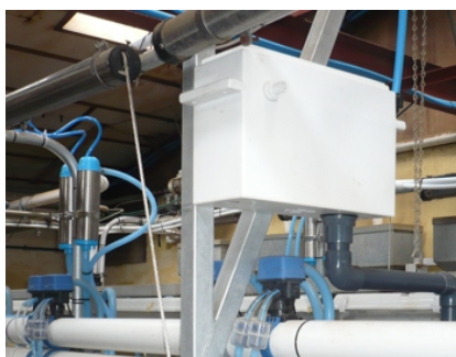
HEADER TANK (Note: Level With Cylinders)
